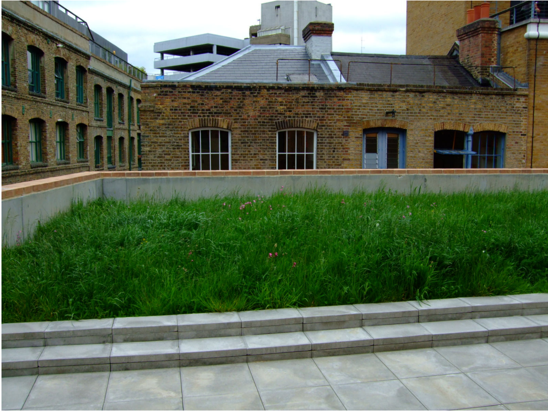
Larger of the two roof terraces, adjacent to the corner of Christina Street and Motley Avenue
