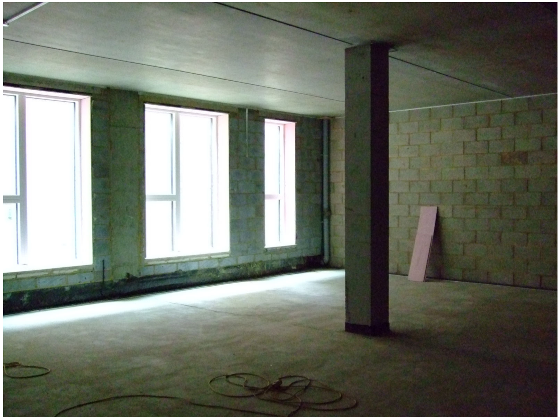
Basement use-class B1 space, showing a lightwell
